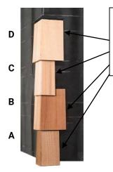
Caulk all butt joints along the cut edge of the panel's plywood backer. Fit snugly against corner pieces, trim, gable edges, window or door trim, etc.
